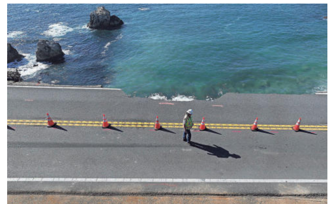
A section of California's famed Highway 1 broke off and fell in the ocean near Big Sur after a heavy storm in March. The road offers amazing views of the Pacific Ocean. JUSTIN SULLIVAN/GETTY IMAGES
