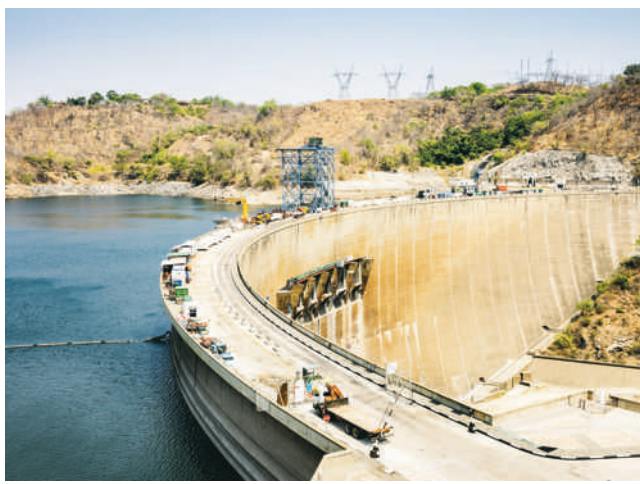
Water levels are so low in the Kariba Dam that Zambia's hydropower plant is operating at one-tenth of its capacity.
